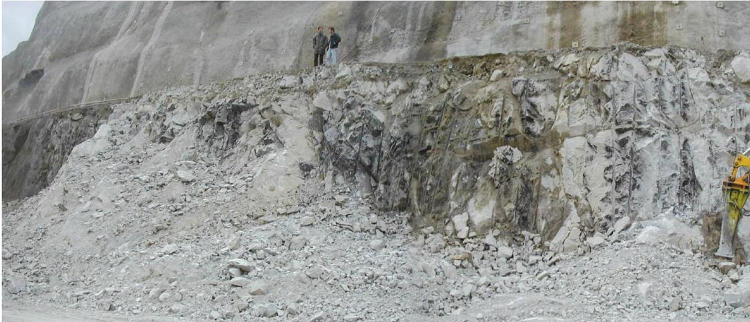
general method used to study the local stability is based on the limit equilibrium of three-dimensional rock wedges bound by two joints. Local stability generally induces a light supporting system on almost every berm, with passive anchors (rockbolts), weld mesh and shotcrete.
