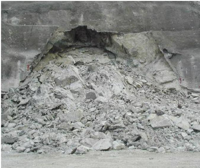
**Left: Fig 8 – Landslide from 2 September 2002 with 300-400m<sup>3</sup> of rock.
