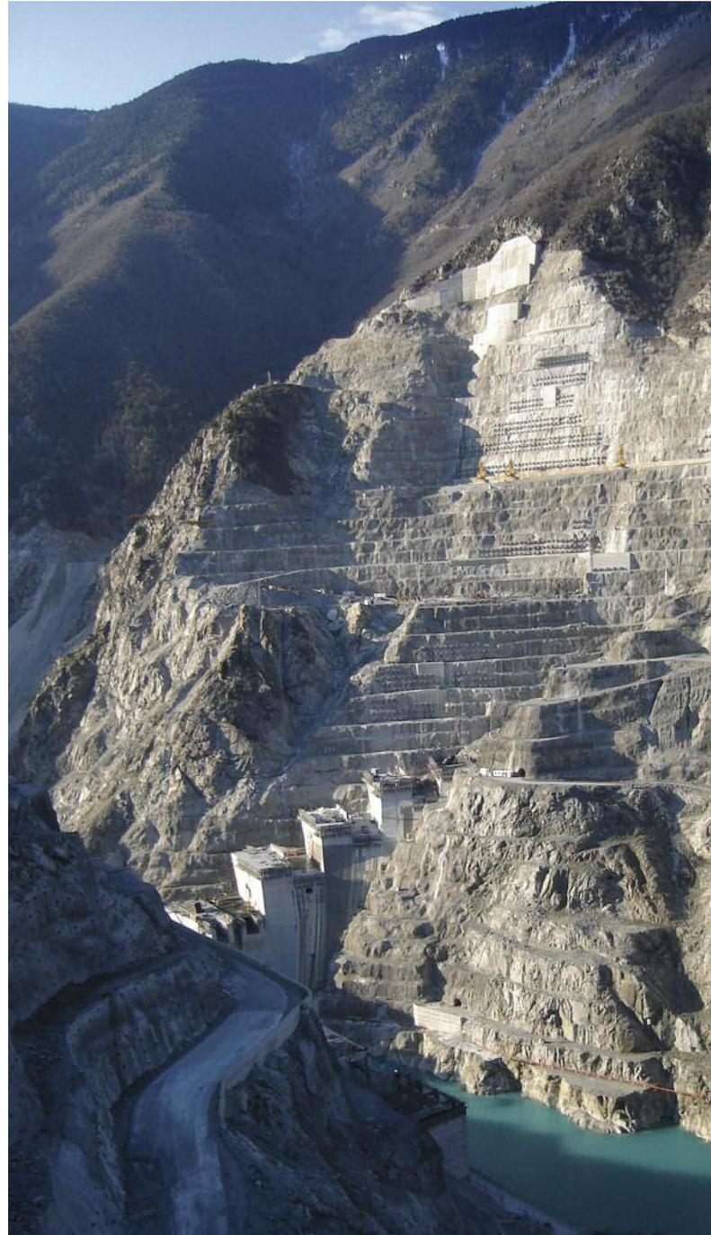
a pre-stressed anchor amounts to more than 5%, additional lift-off tests are undertaken and an updated stability analysis is performed, taking into account all other geological and geotechnical parameters, as well as the continuous monitoring results.
