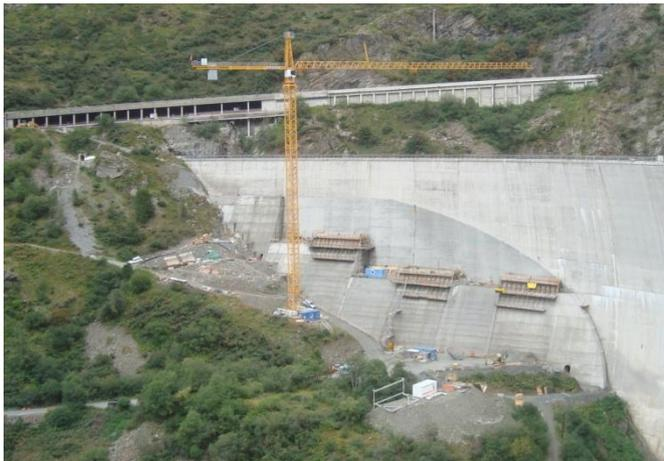
Figure 5: General view of the crane and strengthening work in the right bank (2009)
