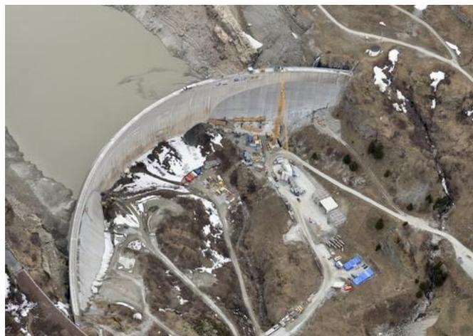
Figure 9: Aerial view of the dam during strengthening works
