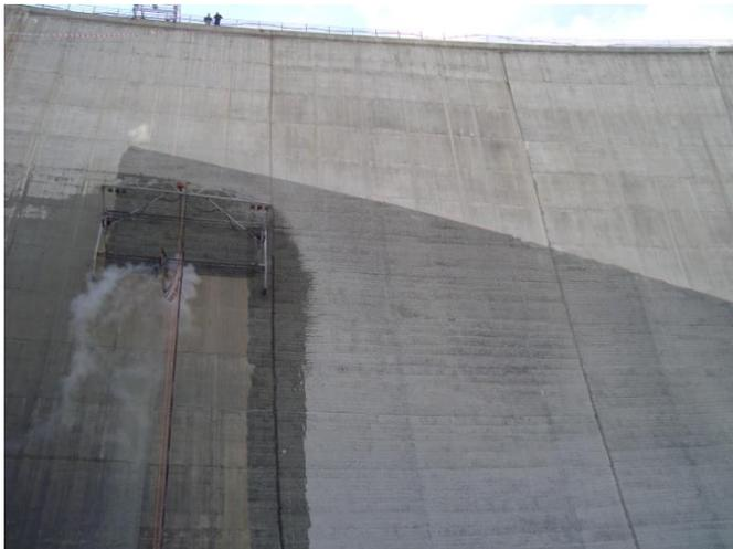
Figure 6: Hydrodemolition as a means to prepare the interface surface between old and new concrete
