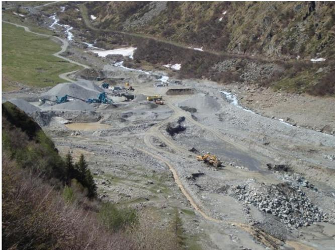
Figure 4: Quarrying inside the reservoir lowered during construction works
