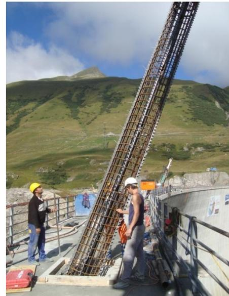
Figure 7: Placing of reinforcing cage after drilling of 700 mm column and before self compacting concrete pouring
